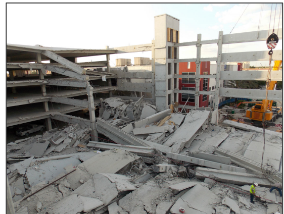
Unmanned Aircraft Systems (UAS) gather information from difficult or dangerous sites.
