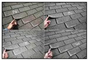
**Figure 16.** Roof in Norman, OK where overlaps were not bonded to the underlying shingles on each directional slope (indicated). This condition was not wind-caused.
