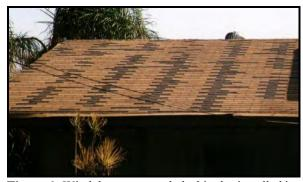
**Figure 6.** Wind damage to asphalt shingles installed in the racking or "straight-up" pattern after Hurricane Frances.
