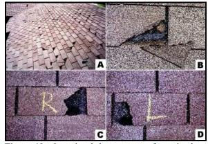
**Figure 19.** Intentional damage to roofs to simulate wind damage: a) broken corners upslope away from roof edge, b) broken corner left nearby, c) torn right edge of tab, and d) torn left edge of tab.
