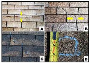
**Figure 14.** Examples of shingle splitting: a) horizontal, b) vertical, c) curved, and d) rounded. Such splitting is not caused by wind.
