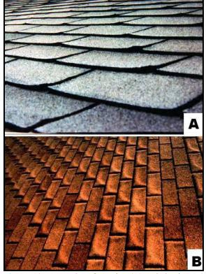
**Figure 13.** Examples of cupping (A) and clawing (B) of asphalt shingles. These conditions are not caused by storm effects.
