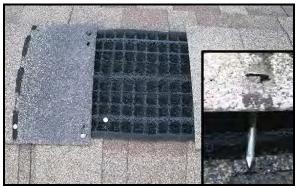
**Figure 12.** Loss of ridge tabs due to insufficient fastener length (inset).
