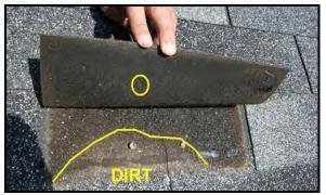
**Figure 11.** Elevated nail (note shadow) prevented this tab from bonding to the sealant strip. Note the dirt residue and smooth sealant on the underlying shingle and lack of sealant transfer to the bottom side of the overlying tab. The yellow circle highlights the indentation of the nail head in the bottom of the overlying tab.
