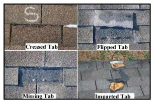
**Figure 7.** Various types of wind damage to asphalt shingles.
