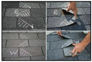
**Figure 18.** Roof in Minneapolis, MN where overlaps were not bonded to the underlying shingles on directional slopes (indicated). This phenomenon was not wind-caused.
