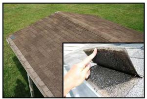
**Figure 10.** Loss of first tab course from Hurricane Ike as the tabs were not sealed down due to improper installation of the starter shingles as shown by inset.
