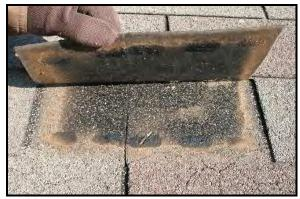
**Figure 8.** This aged tab had little sealant bond strength and could be easily lifted by hand. Note the crazed cracks on the shingle surface.
