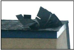
**Figure 2.** Uplift of asphalt shingles on the corner of a gable roof during Hurricane Gustav. Image by Tim Marshall.
