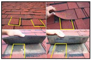
**Figure 9.** Rectangular tabs (outlined) adhered to the tops of the shingles prevented full contact of the overlying tabs and created air gaps between the tabs.
