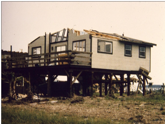
FIGURE 2. Roof shingle and decking damage (left) and severe damage including walls (right).
