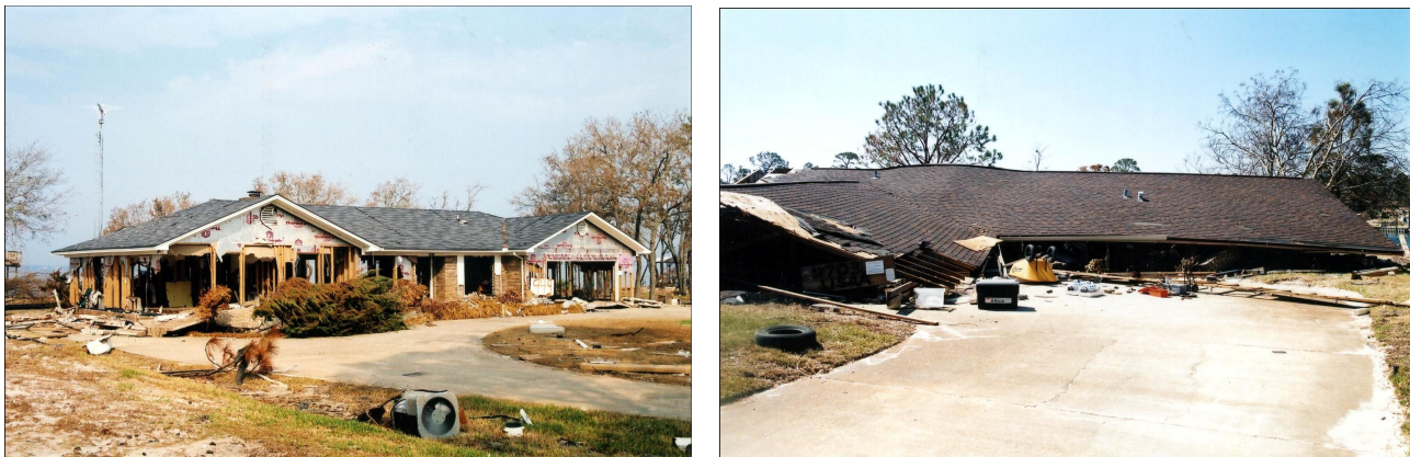
FIGURE 1. Classic flood damage showing washthrough (left) and collapse with no shingle damage (right).
