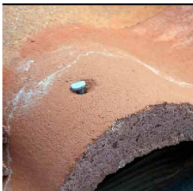
Figure 1: Correct Nail Fastener Installation
