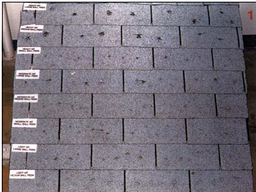
Photograph 1: Composition shingle roof panel
