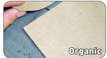
Organic shingles are used more commonly in colder climates. Their increased weight and stiffness help keep them in place in high winds when there isn't enough heat to activate the sealant strips. Organic shingles are less common. "Organic" is included on the "4/09" Shingle Gauge™, but is not on the "01/12" Shingle Gauge™.
