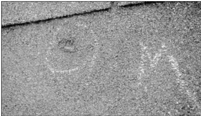
Figure 4. Marring of a composition shingle surface from mechanical abuse.
