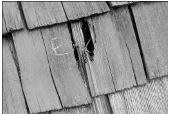
Figure 8. Eroded opening in a cedar shake.
