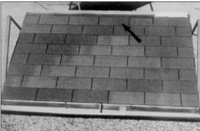
Photo B1. View of test panel at Year 0. Note Tab A-4 at arrow.
